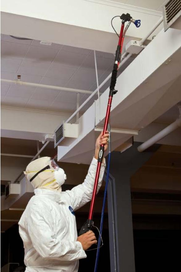
*A spray painting system that lets you spray nonstop, switching easily from gun to pole as you paint. Unlike most poles, the HYDE® RVT™ telescopes-extending your reach up to 12' with no ladders or scaffolding. You'll get faster paint jobs with less fatigue and easy clean-up.*
